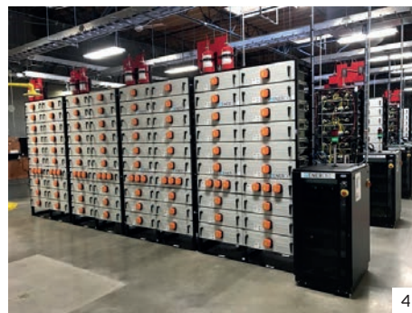
3. EnerDel's 21kWh Vigor+ pack 4. A 1.25MWh Secure+ Grid Energy Storage System
